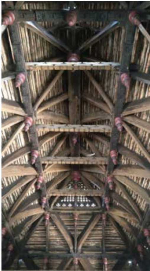
Fig. 4. Wooden roofing at Haripad Temple (Kuthambalam)
