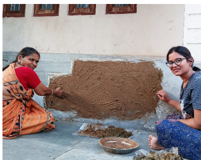
Photo 11: Creating a Wall of Mandana at Home using the Traditional Method of leepan *
