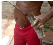
Plate 7: Oiling of Prop Pipe with clay recipe
